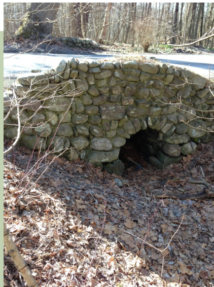
Left. The stone tunnel where water flowed into the mill pond on the east side of the access road.
